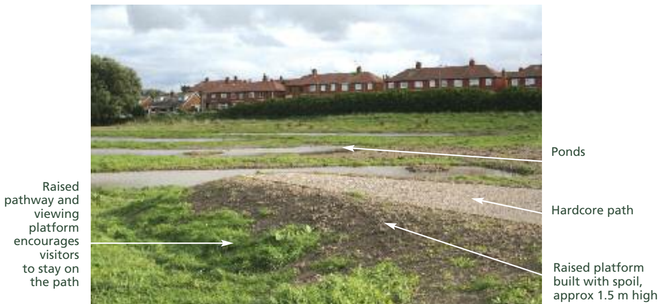
Figure 6. Spoil used to create raised walkway and viewing platform at Lawson's Wetland, Blackpool.
