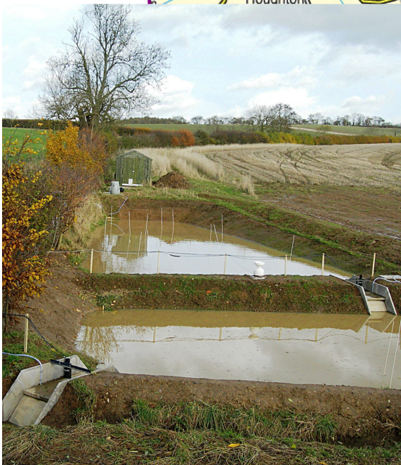
Phosphorus and sediment trapping ponds at Loddington. These ponds are part of the Defra funded MOPS project
